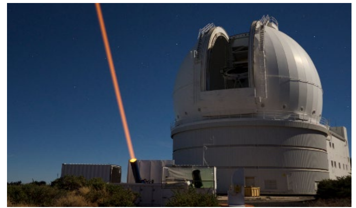
WLGSU in operation outside the WHT
